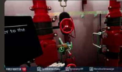
Sprinkler System Maintenance
